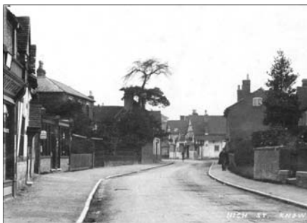
Left: High Street looking towards the church..
